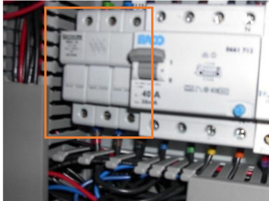
Figure 2 - 3-phase fuse holder
